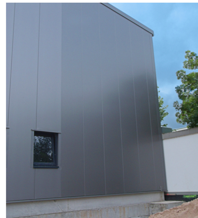
Unintentional colour changes between foamed and stone wool sandwich panels
