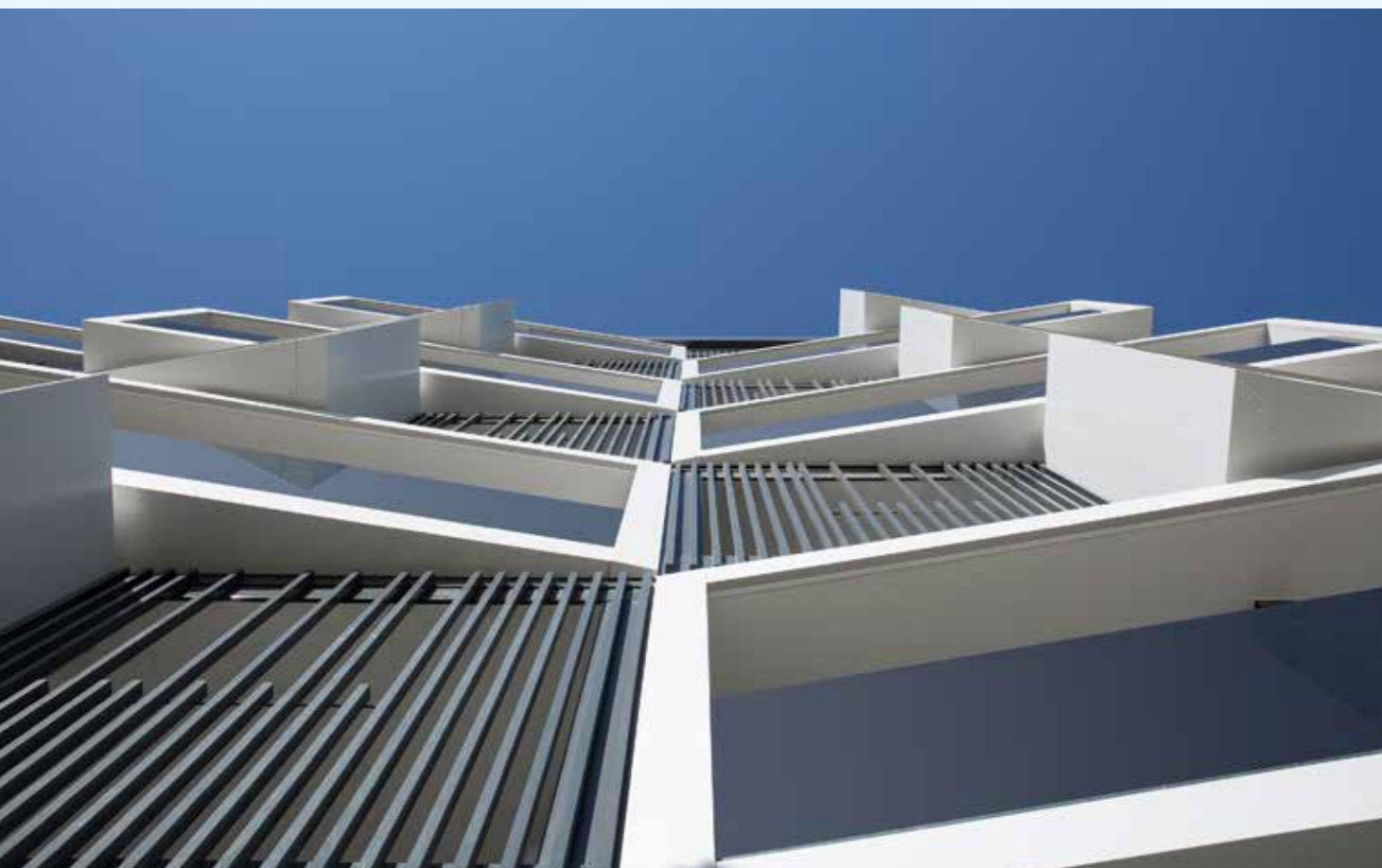
Pamplona, Spain. Products: Ventirock Duo | REDair insulation
