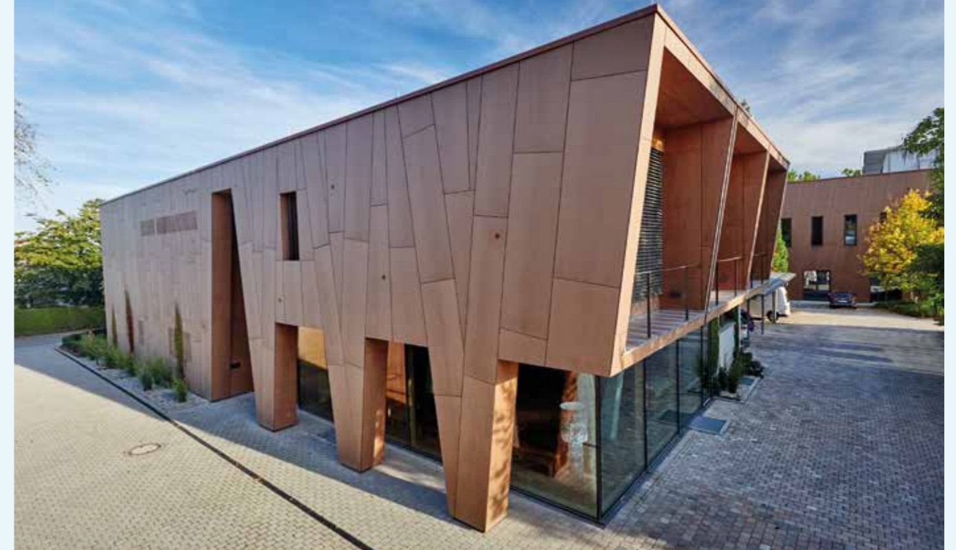
Eggenfelden, Germany. Products: Rockpanel boards | Rockclad boards (RAL 7016) | ROCKWOOL Fixrock
