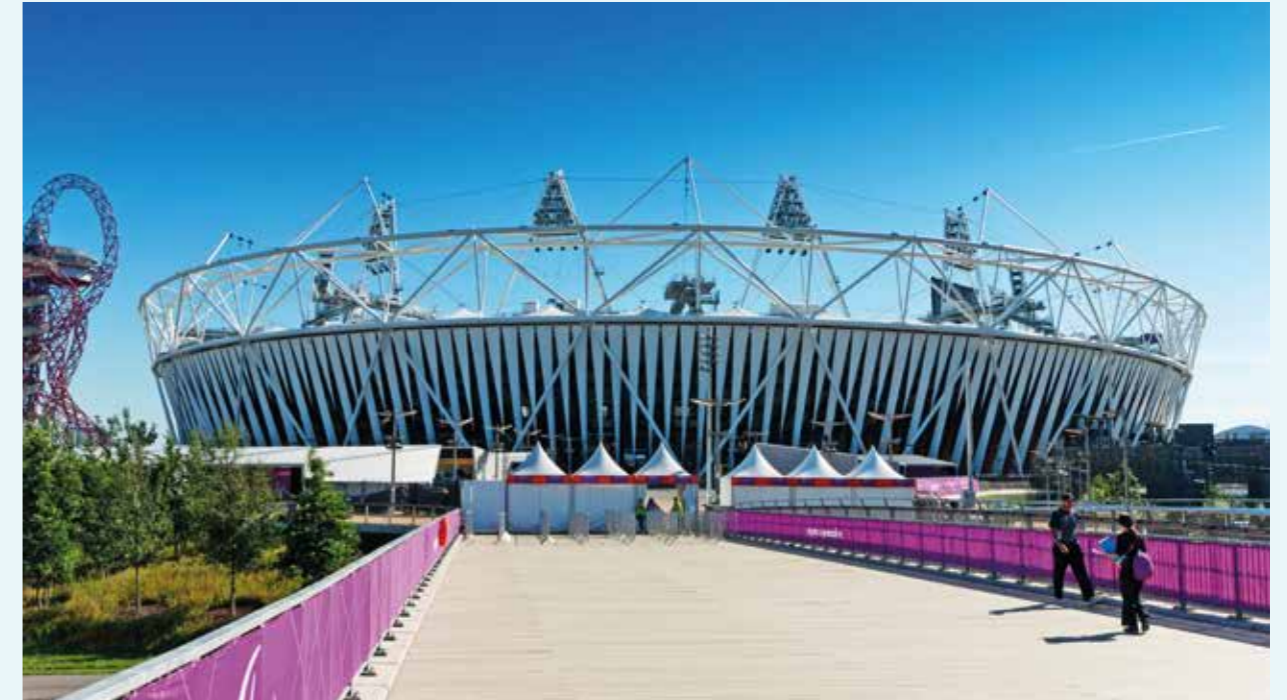
London, UK. Products: ROCKWOOL HARDROCK® Multi-Fix | ROCKWOOL Acoustic Infills
