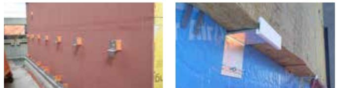
Examples of thermally improved discrete cladding supports for composite metal panels.
