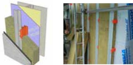
Fiberglass clips with vertical Z-girt attached to wall with screw fasteners through the fiberglass clips into the back-up wall.
