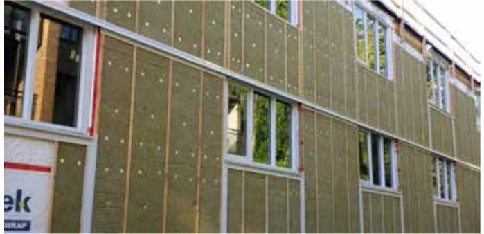
Example of insulation retained by mechanically attached impaling pins between vertical wood framing (adhesive stick-pins are not considered a long-term support strategy).
