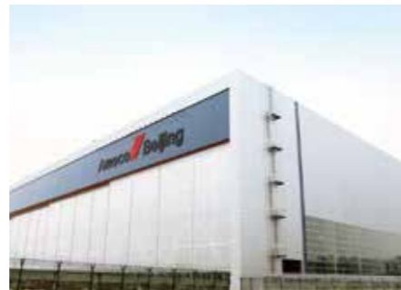
A380 Hangar, Beijing Capital International Airport, China
