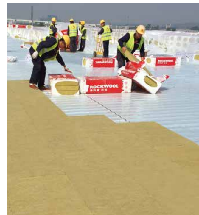
China Aviation Lithium Battery Co.,Ltd Project (Zhengzhou)
