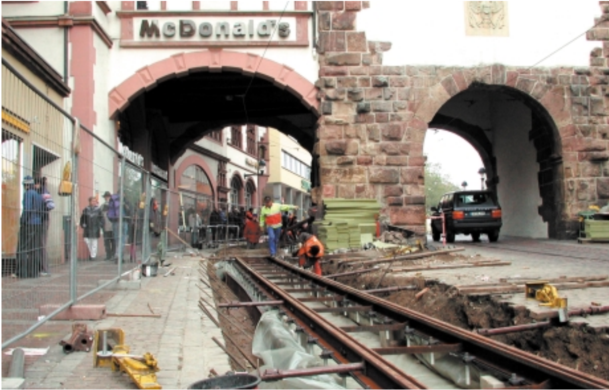
RockDelta a/s was established in 1997 to sell green sound barriers for e.g. road noise and vibration boards for railway tracks. The picture shows vibration boards used in the old town of Freiburg, Germany.
