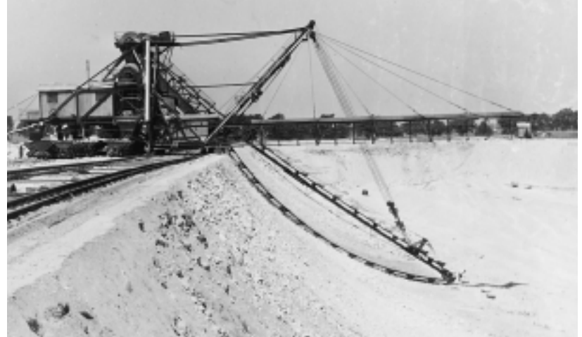
The bucket-ladder-excavator at Nymølle Skærvefabrik, Hedehusene, in 1933 before the insulation business began.
