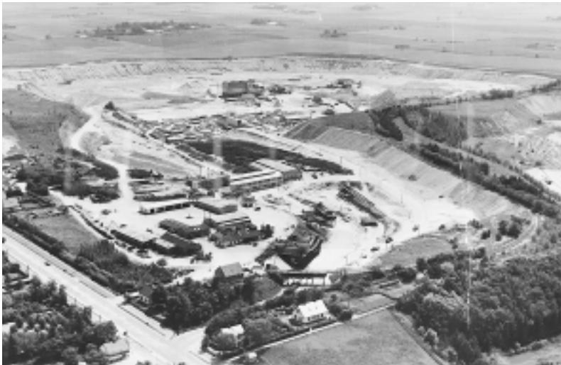
The factory in Hedehusene in 1954. It is placed in a gravel pit.
