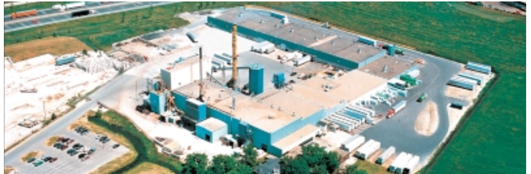
Milton, Canada – the first factory outside Europe, 1988.
