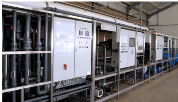
Figure 11. Picture of the technical installations in the water technical room. The setup shown here allows the grower to quickly check the proper functioning of all systems.
