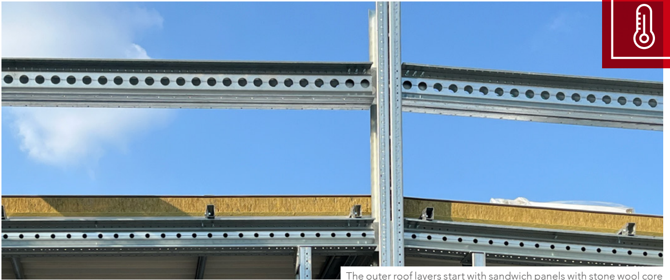
The outer roof layers start with sandwich panels with stone wool core
