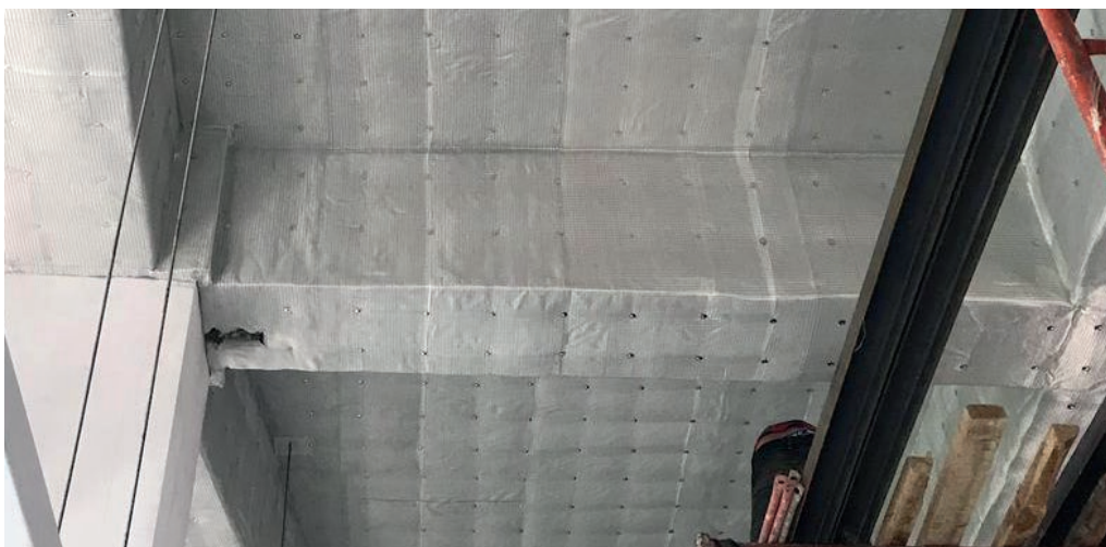
Image 3: Example of beam insulation
